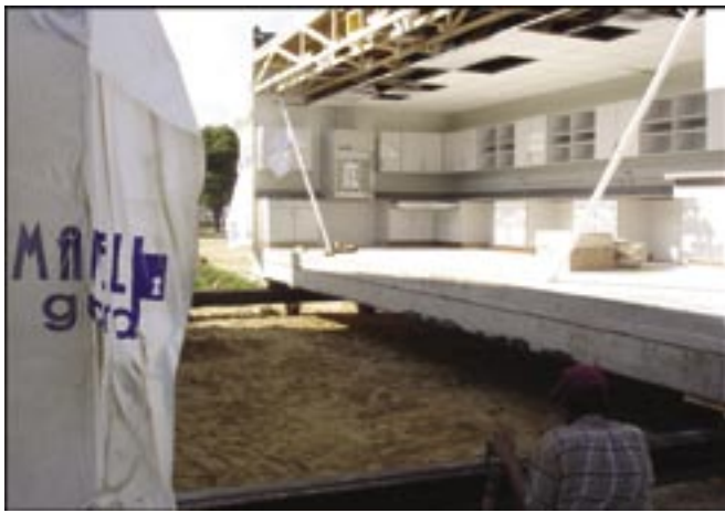
Interior view of the new Navasota, TX High School 1500 sq. ft. science lab classroom. Installed on-site just in three days and ready for classes to begin. All the equipment was pre-installed in-plant saving time during the installation process.
